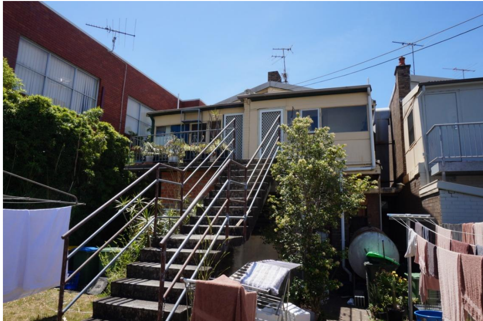
Figure 8 - Rear elevations of the building with later residential access stairs and single storey service outbuildings. Narrow light wells provide light and ventilation between the rear service wings over two floors.
